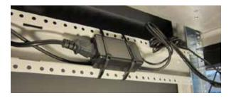
Figure 2 – Radio 12V DC Power Supply
