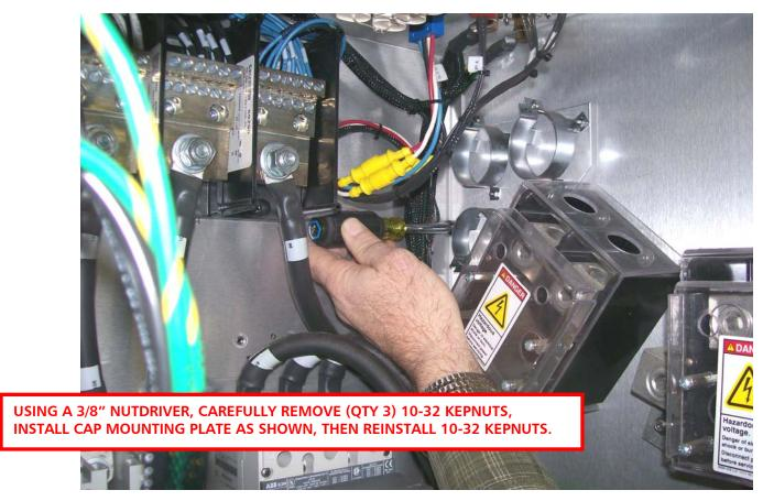
Figure 7 – Install Cap Mounting Plate into 4MX
