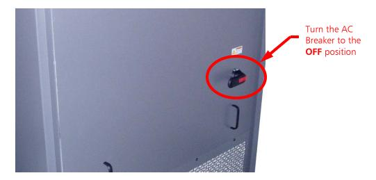
Figure 6 – Turn 4MX AC Breaker to OFF
