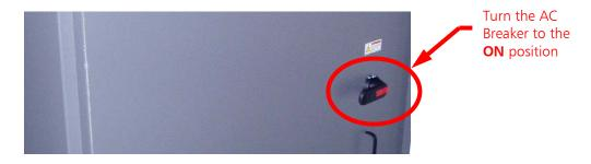
Figure 11 - Turn 4MX AC Breaker to ON
