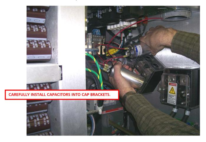
Figure 8 – Install Capacitors
